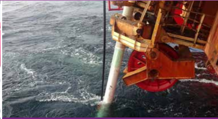
DEH cable and pipeline installation
