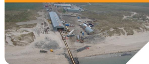
Wick Fabrication Site, UK
