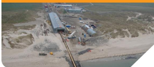
Wick Fabrication Site, UK
