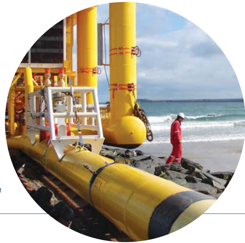
A pipeline Bundle is launched at our Wick fabrication site
