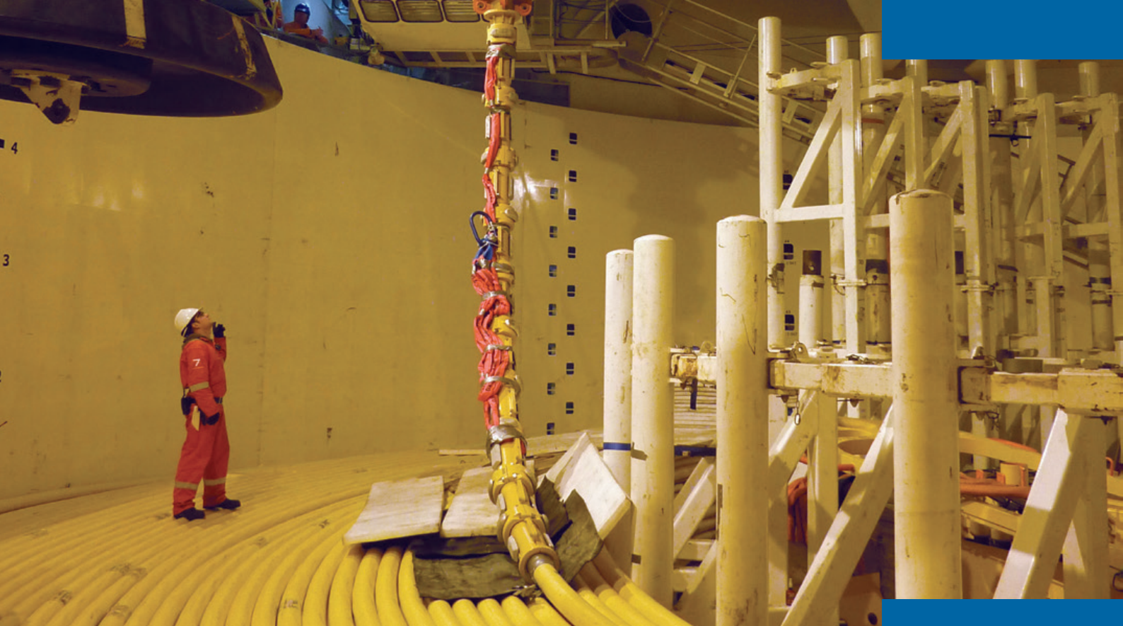
Umbilical Loadout on Skandi Acergy
