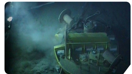
Pipe-walking chain installation by Simar Esperança
