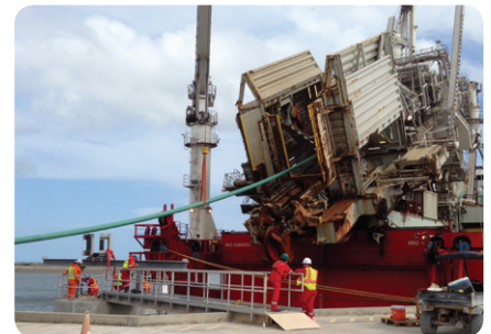
Reeling pipe onto Seven Oceans
