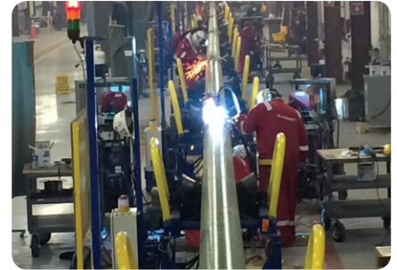
Fabrication of pipe-in-pipe at Port Isabel Spoolbase
