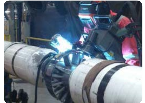
Welding at Ubu Spoolbase
