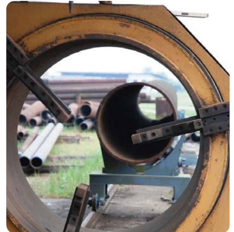
Fabrication at Warri yard
