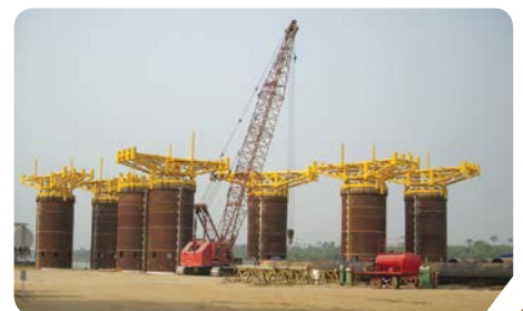
Piles fabrication at Warri yard
