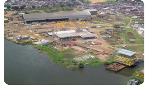
Aerial view of Warri yard
