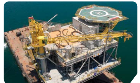
Mafumeira Topside in Lobito yard
