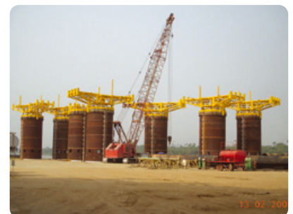
Fabrication at Warri Globestar Yard
