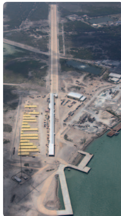
Aerial view of Port Isabel Spoolbase
