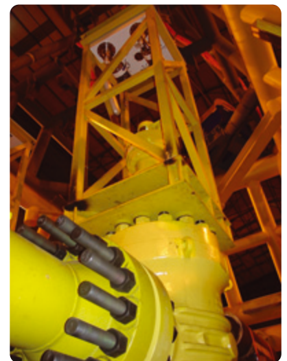
The preparation and execution of a Subsea Hot Tap
