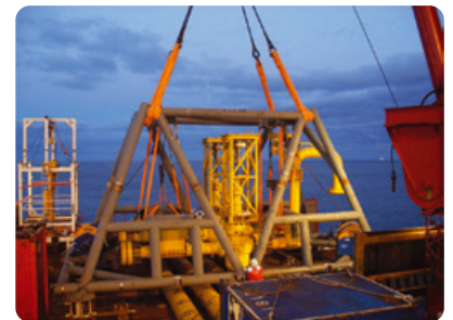
The preparation and execution of a Subsea Hot Tap
