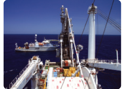
Seven Oceans laying pipe and Seisranger performing touch-down monitoring
