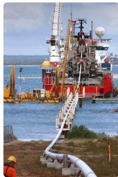
Spooling onto Seven Navica at Crib Point
