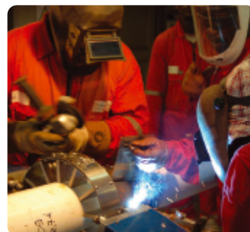
Angolan Welders fabricating flowline stalk at Luanda spoolbase
