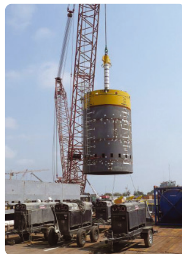
Suction pile for production manifold
