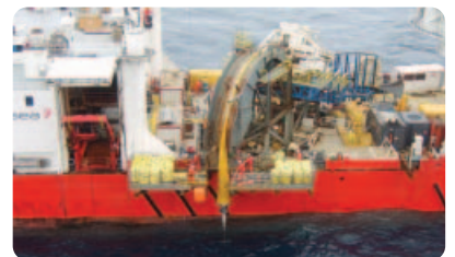
Umbilical installation by the Skandi Neptune
