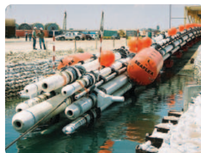
Riser tower bundle assembled at the Sonamet Yard in Lobito
