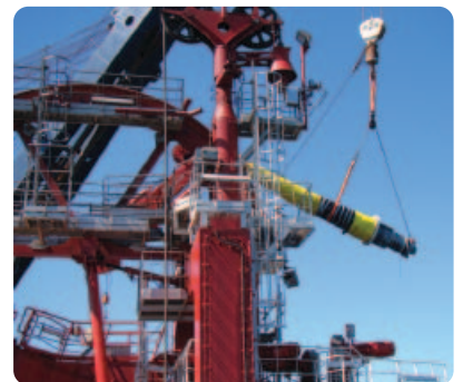
The Toisa Proteus Flowline installation
