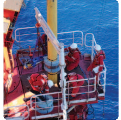
The Toisa Proteus Flowline installation
