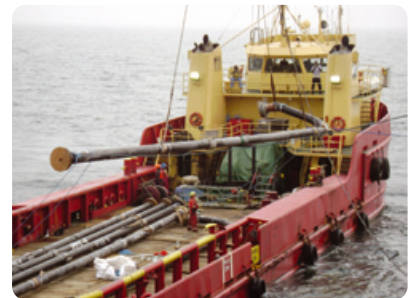
Installation of 12 inch tie-in spool
