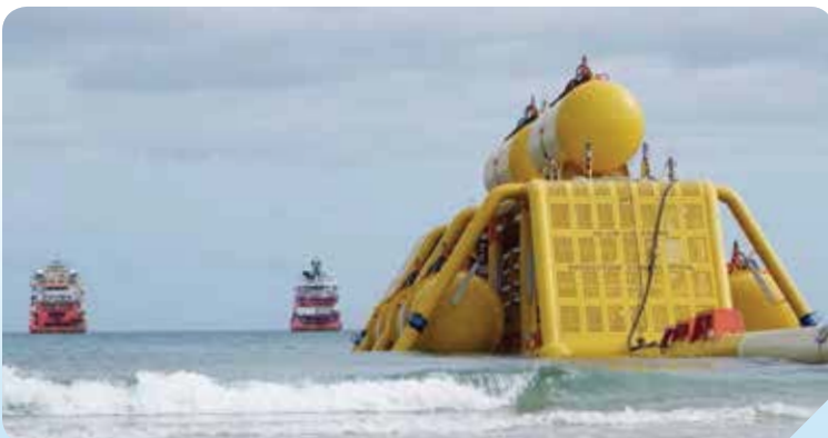
Launching an advanced pipeline Bundle at Wick, Scotland, for the Knarr project in Norway
