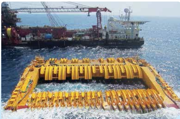
One of the four Buoy-Supported Risers (BSRs) now installed and operational on the Guar-Lula NE SURF project in Brazil
