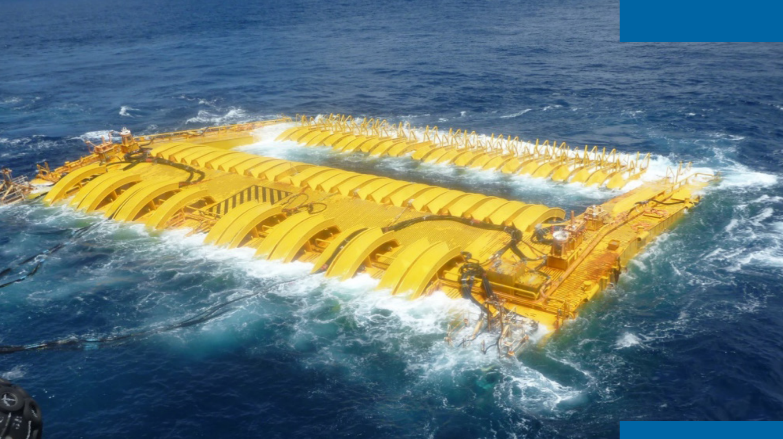
Buoy-Supported Riser in location, ready to be submerged and installed
