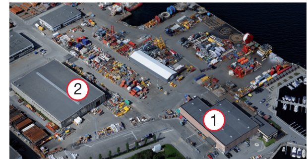
Dusavik Base Overview 1 - Warehouse/Workshop 2 - Warehouse
